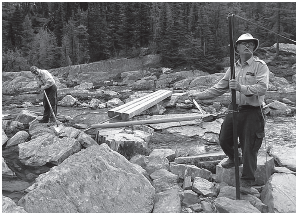
Parks Canada trail crew workers Matt Cadden (l) and John Morrison (r) use a "come-along" to move a large rock into place on the Opabin Plateau.
